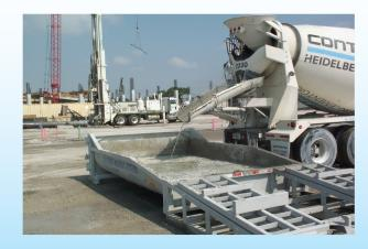
The use of concrete washout bins is noted by the EPA as a Best Management Practice. The EPA states, "Wash water is alkaline (very high ph level) and contains high levels of chromium, which can leach into the ground and contaminate ground water." The EPA also states, "When selecting a company to handle concrete waste, ensure that they are properly disposing of <u>ALL MATERIALS</u> and give preference to companies that recycle collected materials."
